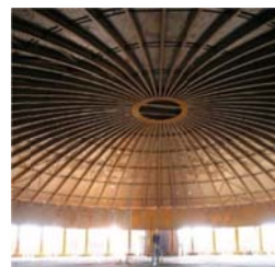
Storage tanks at Andasol 1
